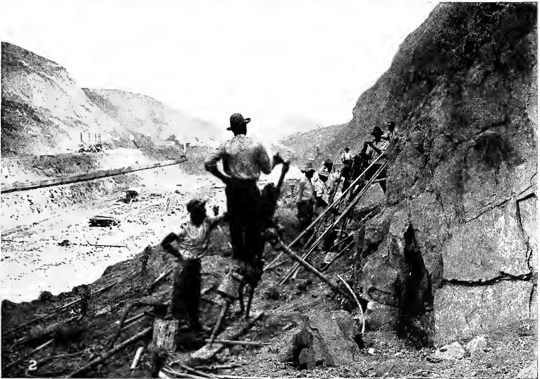
1. Battery of well drills at work in foreground and another in the background, preparing for a gigantic blast. 2. Battery of tripod drills at work.
