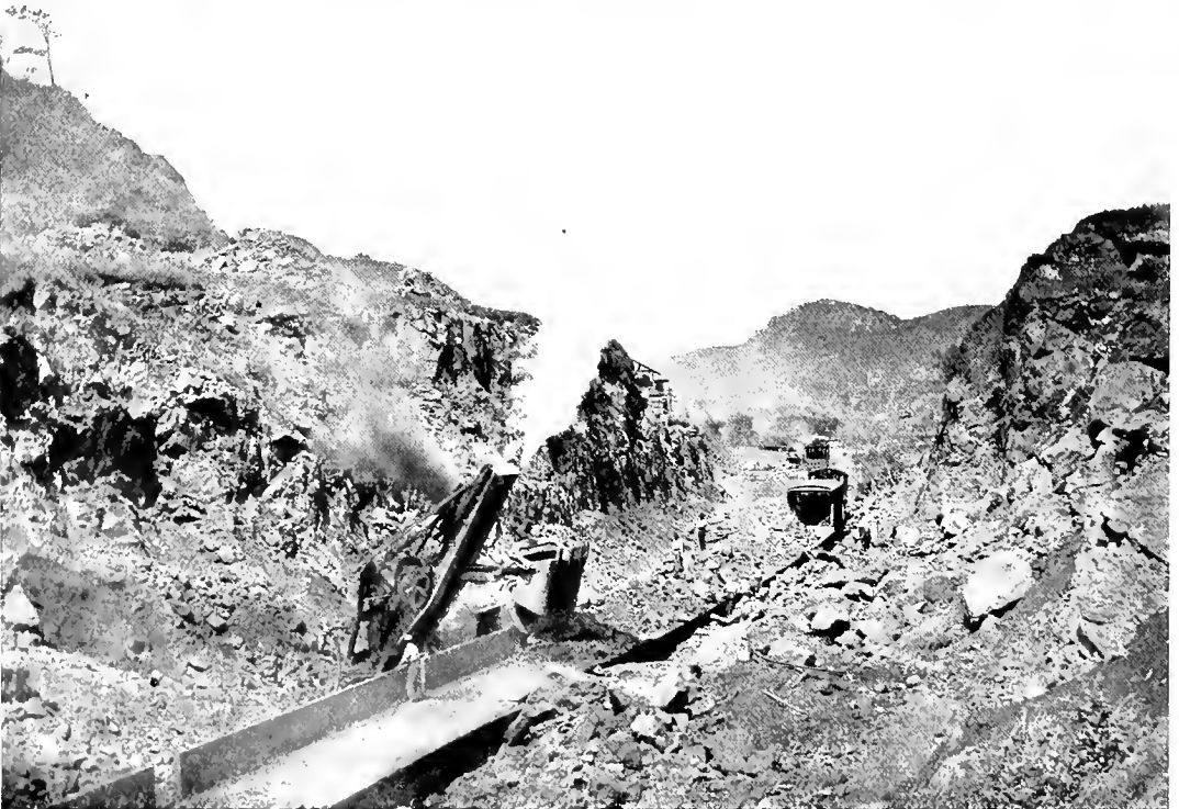
1. Steam drills at work preparing for blasting. 2. Steam shovel loading a Lidgerwood train, 1906.
